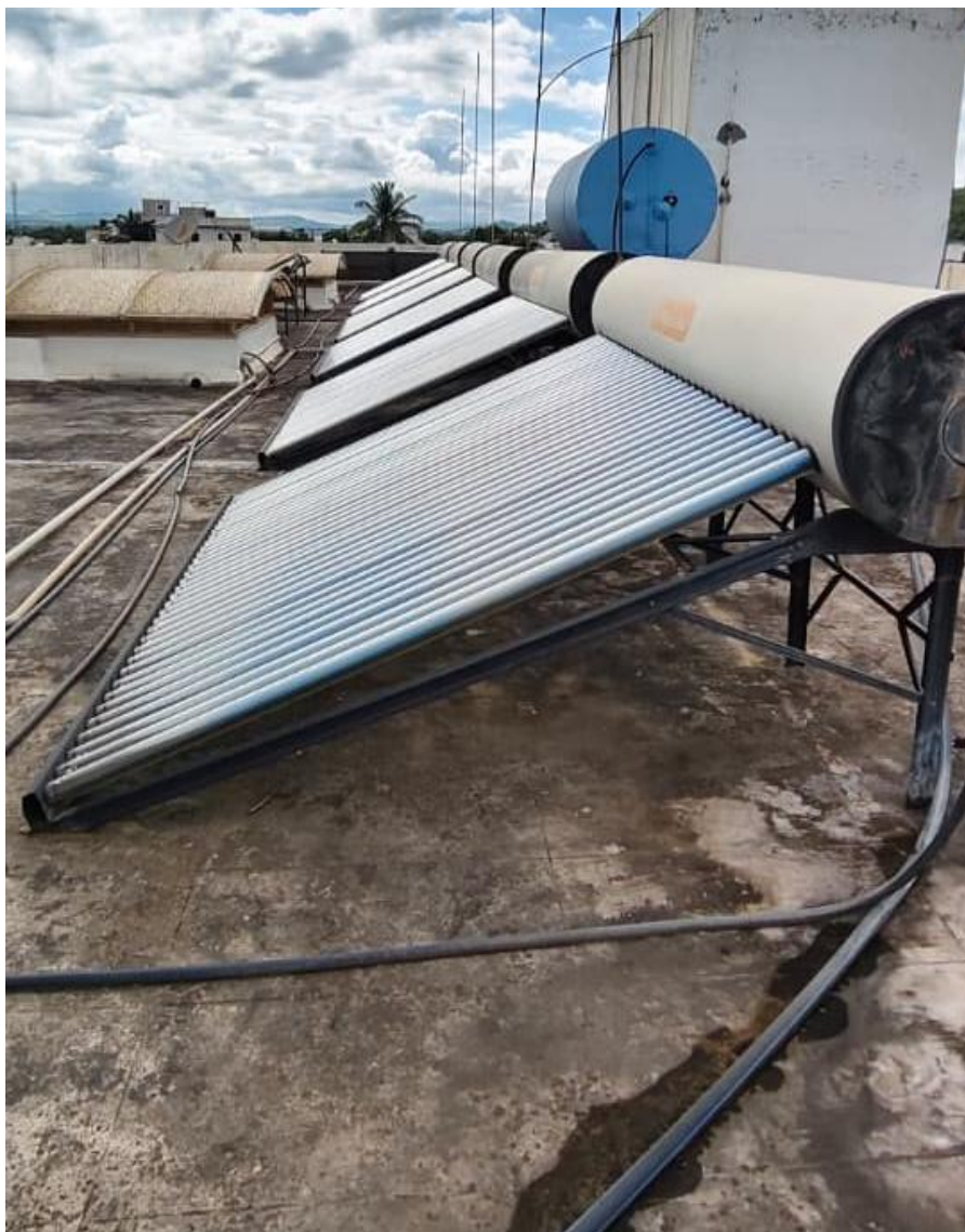
Photo-3: Solar water heaters on Seth Govind Raghunath Sable College of Pharmacy building
